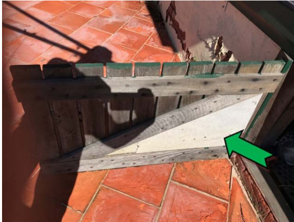
Photo 1. Exterior, store, door panel – non asbestos-containing fibre cement sheeting.
