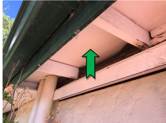
Photo 2. Exterior, throughout, eaves – non asbestos-containing fibre cement sheeting.
